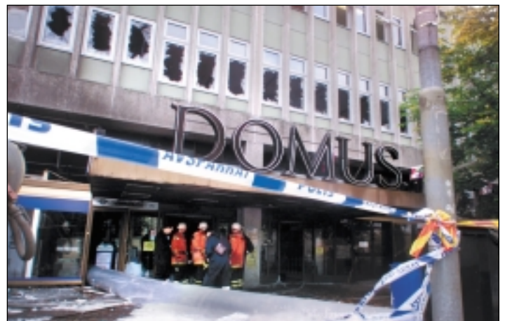
The complete streetfloor was destroyed in the fire
