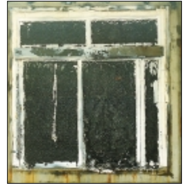
Sliding Door - exposed side after 60 minutes test
